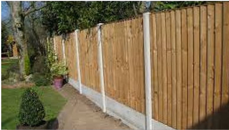
Concrete Post & Wooden Panel Fence
