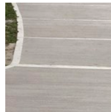
Brushed Concrete with trowel edge finish (streets)
