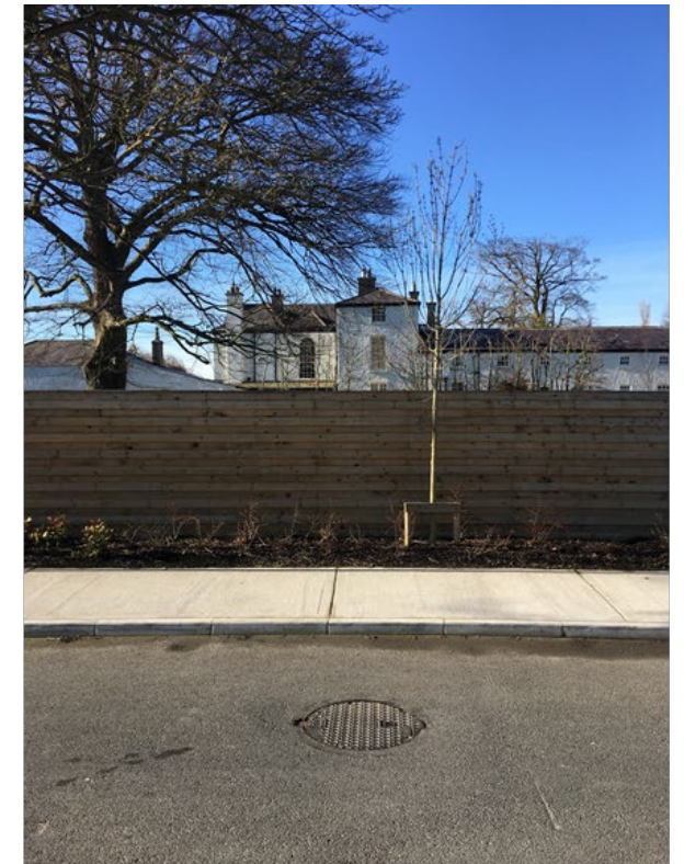
Double Sided Treated Wooden Panel Fence With internal concrete post & Gravel Board
